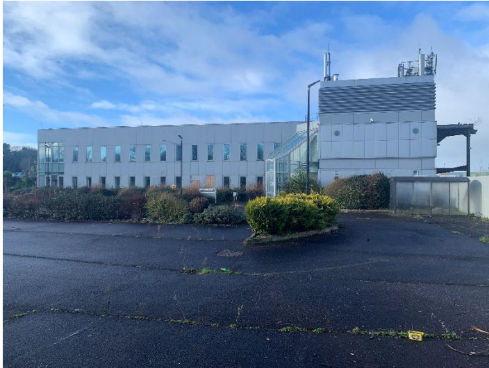
Plate 3-1: Former Dell building constructed of sheeting with no suitable habitat for nesting birds or roosting bats
