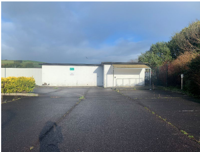
Plate 3-2: Flat roof building at the north-east of the site
